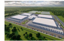
A rendering of the data center campus, commonly known as the First StarGate Project, in Abilene, Texas, being developed by Crest Energy.
